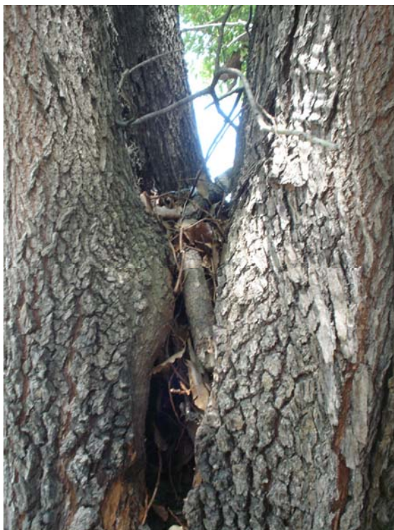
Photograph 3: Tree # 112 – Illustrating the failure and hollow at the junction of codominant trunks at 1.2 metres.
